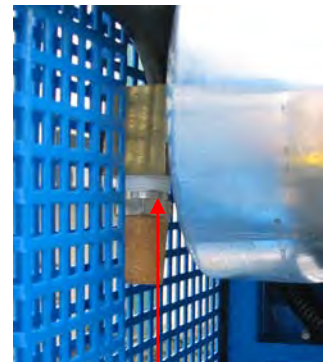
Fixed Factory Set Nitrogen Discharge
